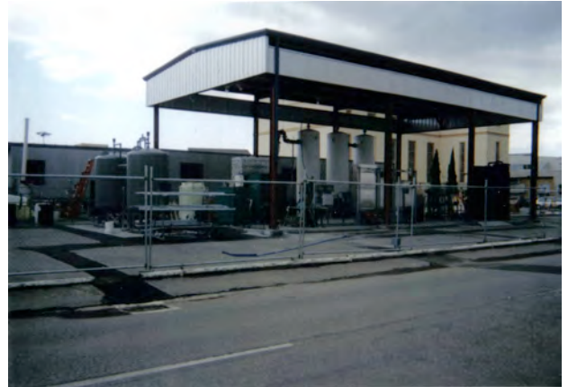
100 GALLON PER MINUTE PUMP AND TREAT SYSTEM NASA AMES RESEARCH CENTER, MOUNTAIN VIEW, CA
