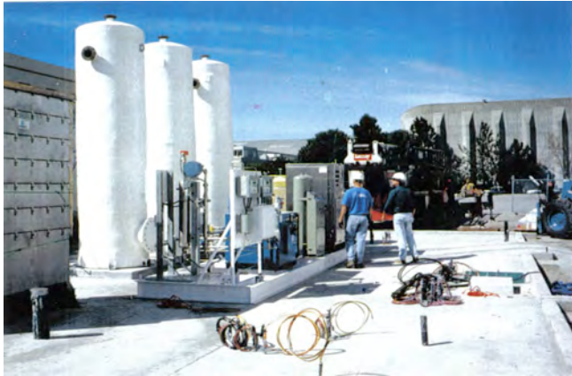
100 GALLON PER MINUTE PUMP AND TREAT SYSTEM NASA AMES RESEARCH CENTER, MOUNTAIN VIEW, CA
